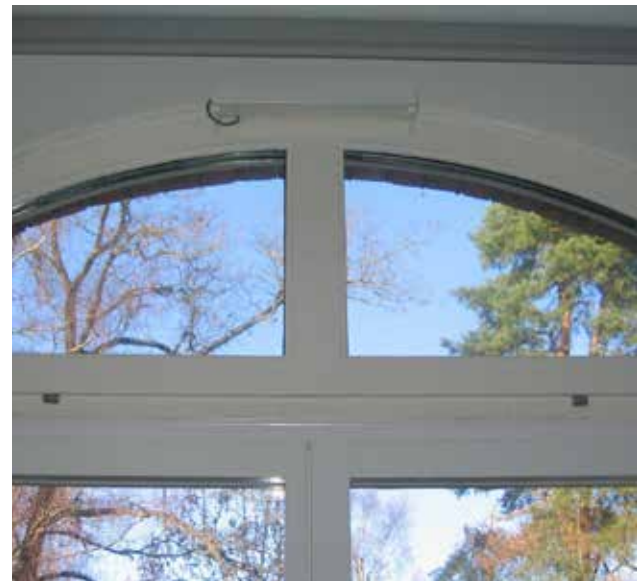
This picture shows an example of how old ventilation windows can be supplemented with a motor.
