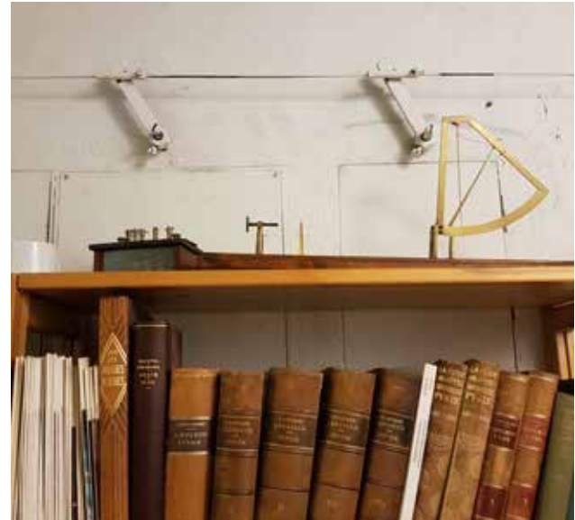
The old dampers were motorised when refurbishing the calorifier system 100 years after the school was originally built.
