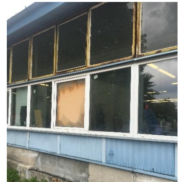
Figure 2: Windows on building 7.
