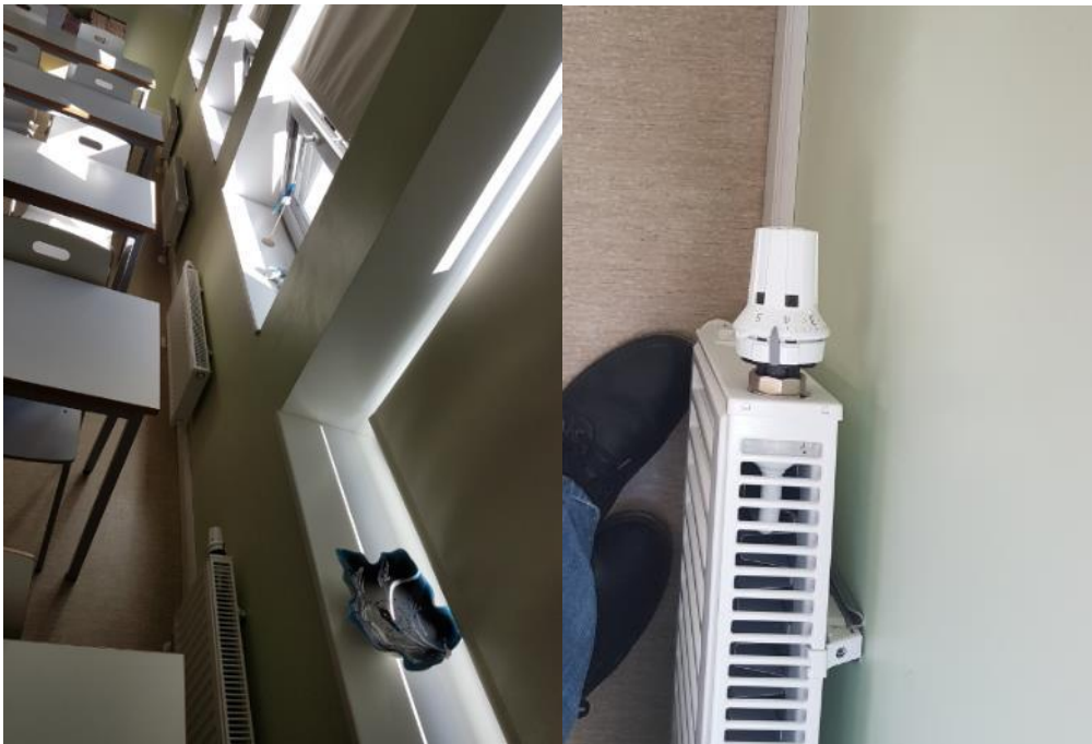
Figure 3. The windows are open due to overheating and the radiators are switched on
