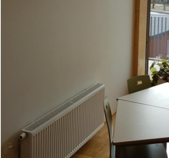
Figure 22. Inappropriate placement of the radiator
