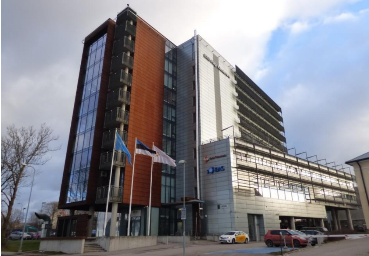
Figure 25. Lasnamäe 2 office building (source: https://www.arihooned.ee/719-lasnamaee-2 )
