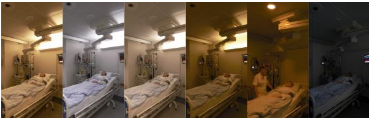
Figure 3: As the day progresses, the natural light emitted by the sun changes in color, angle, and intensity. A circadian lighting system can be designed to mimic that progression. Image taken from Chromaviso (2018a).
